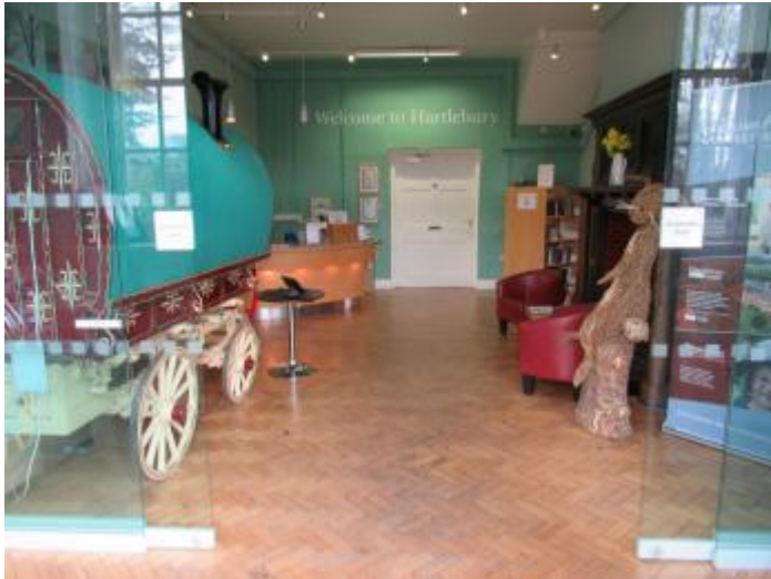
The contrast markings on the glass Reception doors
