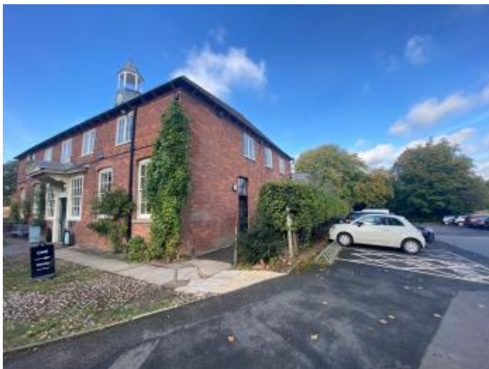
Level access entrance to Reception and Cafe
