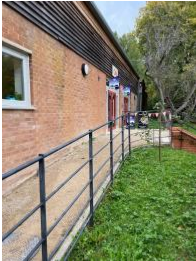
Accessible level access path to Hayley's Kitchen Cafe
